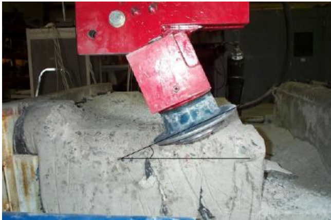
Figure 12 Undercutting with 8” disc on LCM
