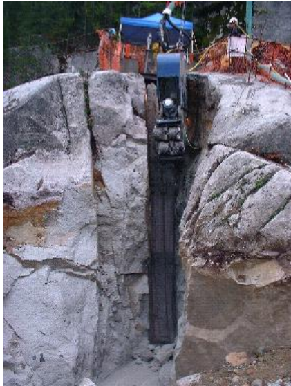
Figure 2 Lowering into position
