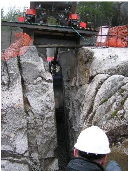
Figure 3 Cutting at quarry
