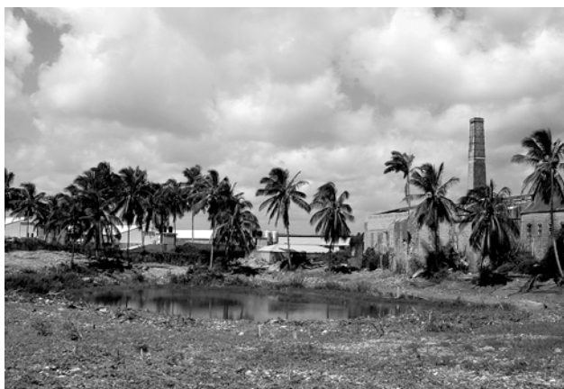
FIGURE 2. Photograph of Pond 3 showing disturbed soils and proximity of mill.
